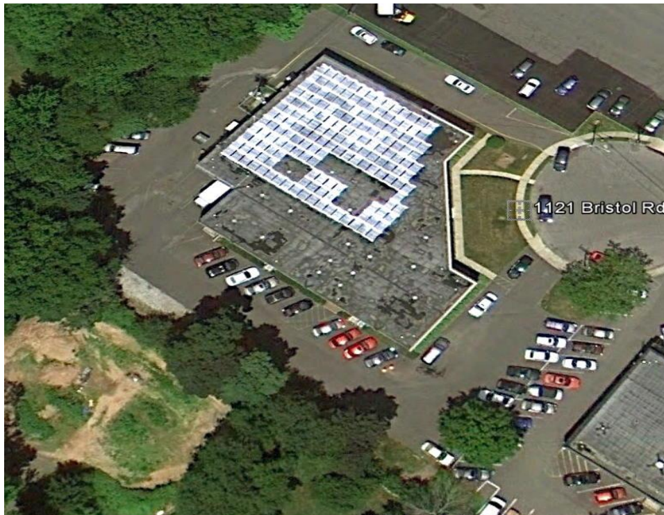
Ariel View-Note Solar cells on Roof
